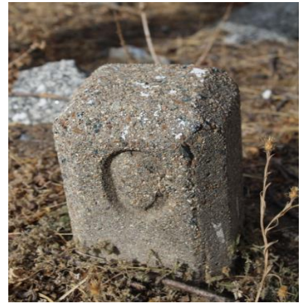
California "C" road markers that pre-date Route 40 can be found in Placer County.
